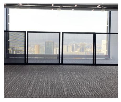
Being more energy-efficient, and providing more cost savings, the new era of green buildings is here to stay. SSG®'s Glass Integrated Photovoltaic (GIPV) is the embedding of silicon solar cells in glass panes and integration of such panels onto buildings for electricity generation.
