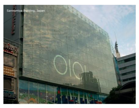
SSG® Concealed Point Glazing (CPG) System is a specially designed proprietary point fixed system that is concealed within the laminated glass façade structure. Traditional structural glazing systems have its point fixing elements designed to flush with the glass surface. However, through the development of technology and materials, it is now possible to have a seamless exterior glass façade with the adoption of the SSG® CPG system.
