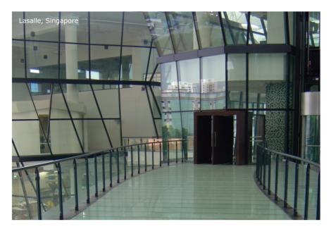
The SSG® SlipResistant provides an ideal solution for slippery glass floors by incorporating a special slip-resistant coating to produce a hardwearing glass surface. It is available in colourless, silk-screen and a translucent colour with a wide range of patterns, allowing architects to get creative in their
