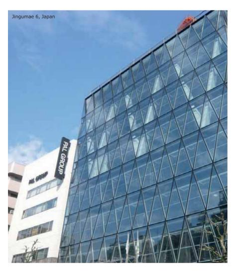
Annealed glass is a brittle material that breaks under low tensile stress. The exposure of annealed glass to wind load or extreme changes in temperature (about 40-50°C) can cause tensile stresses sufficient for annealed glass to break. In overcoming its fragility, a tempering process can be used to increase tensile strength of glass as a structural component.
